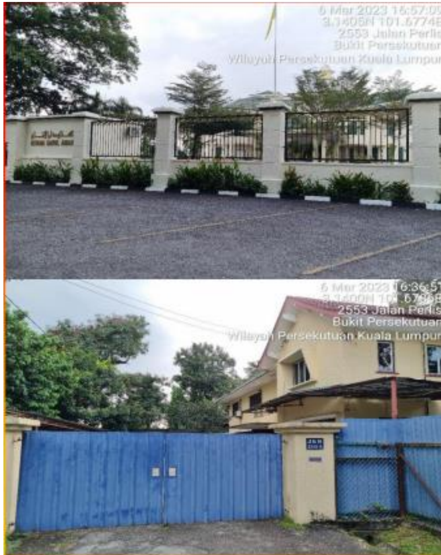
Plate 2.2: Some of the buildings on the contour of 105 to 110 m a.s.l. which forms part of the hilltop of Pulai Trail Urban Community Forest.
